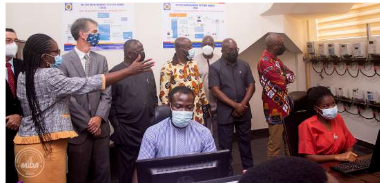
Ing. Sariel Etwire (ECG Project Manager, Meter Management System - MMS) explaining system to Hon. Andrew Egyapa Mercer, Deputy Energy Minister (5th left) and others after MMS inauguration
