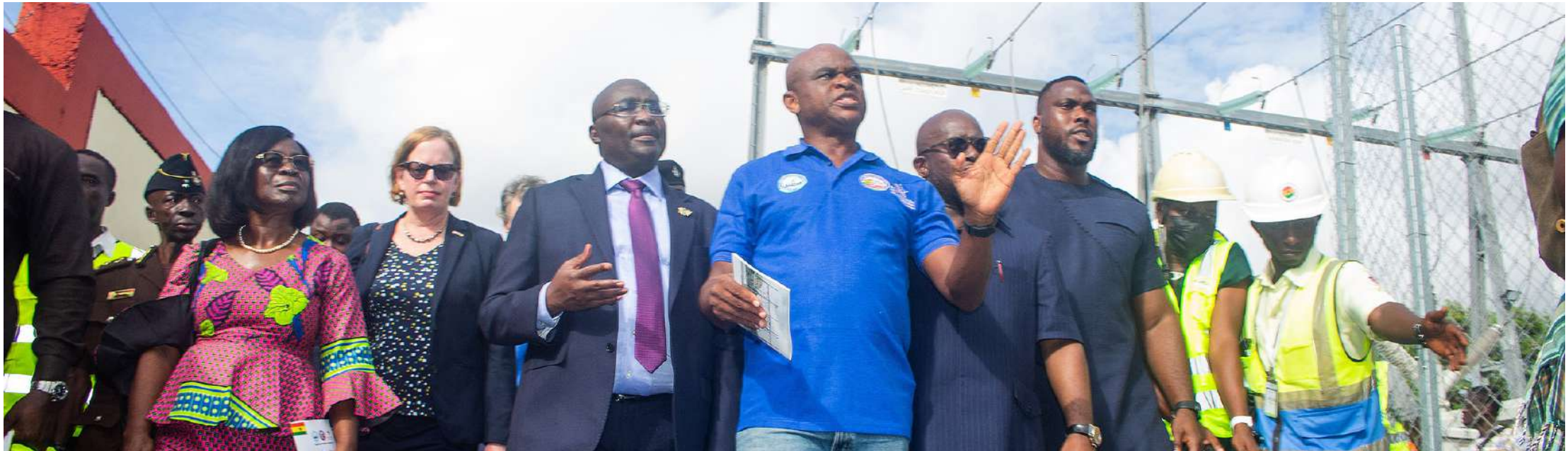
Ing. William Amuna, Technical Controller at MiDA, conducting Vice President Alhaji Dr. Mahamudu Bawumia on a tour around the Kasoa BSP site
