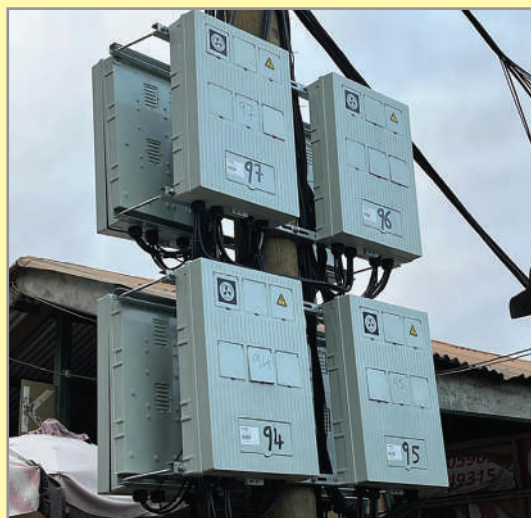
Pole-mounted Meters
